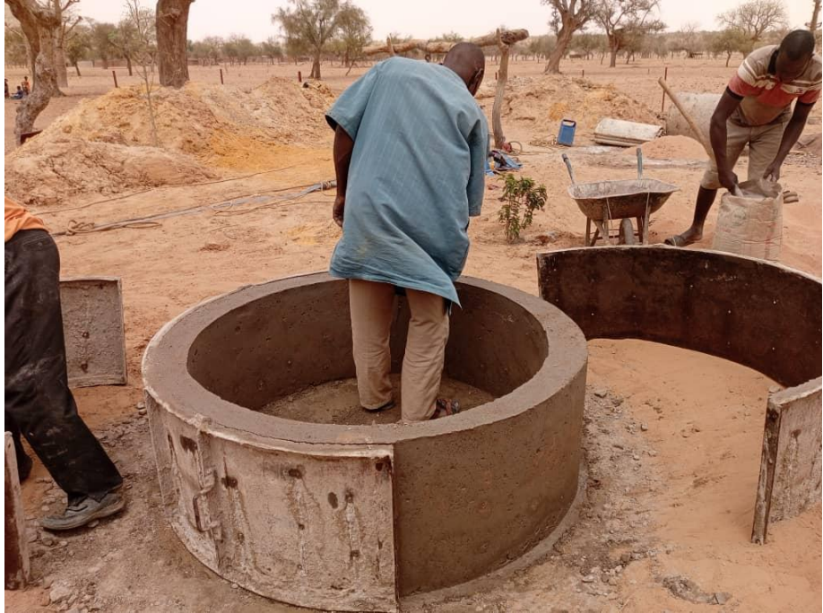
Removing the concrete mold from a section of the well.
